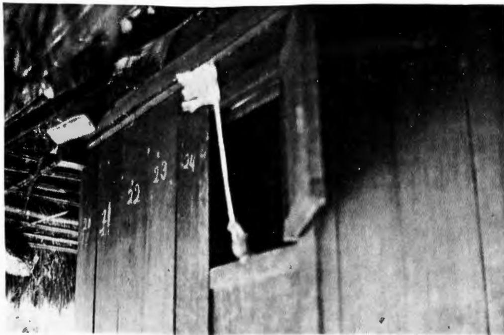
36: House of a deceased woman. The planks are numbered because the house is to be built on a different site after the burial. The whisk is used to keep flies away from the corpse.
